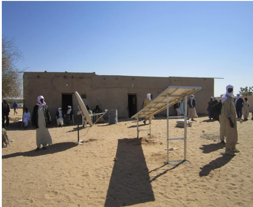
Youth club equipped with solar system to run satellite TV set and provide lighting services
